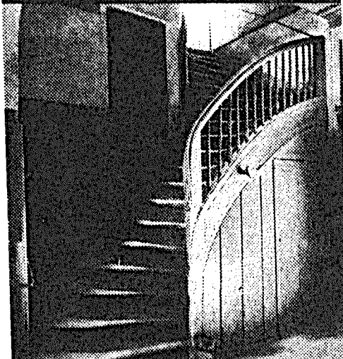
Staircase in a tenement building Landsberger Strasse 1872
